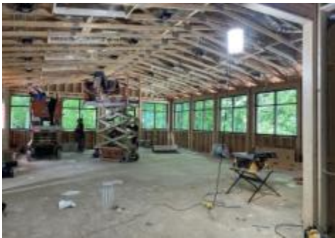
Construction Photos Week of 5/17/2023
