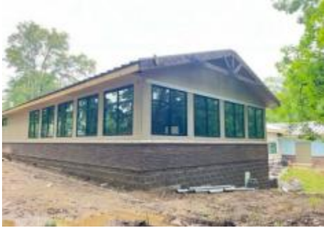
Construction Photos Week of 6/16/2023
