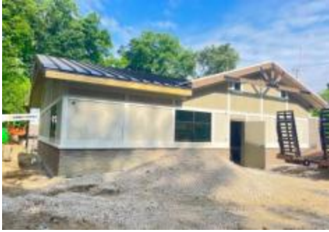
Construction Photos Week of 6/30/2023
