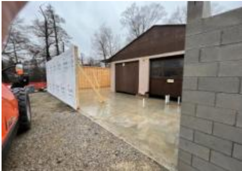
Construction Photos Week of 1/16/23
