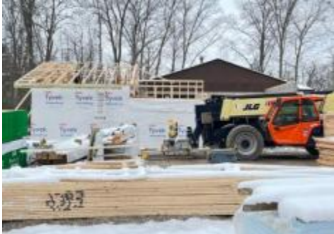
Construction Photos Week of 1/23/23
