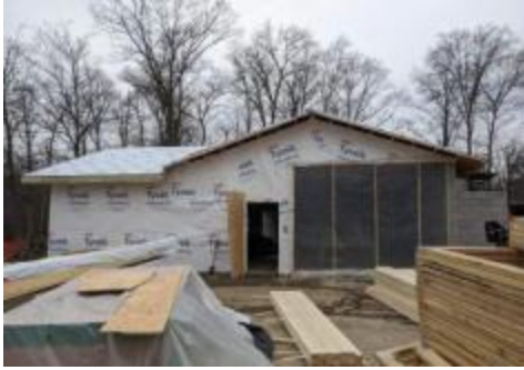
Construction Photos Week of 2/6/2023
