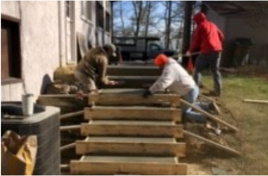
Walk way Improvements
